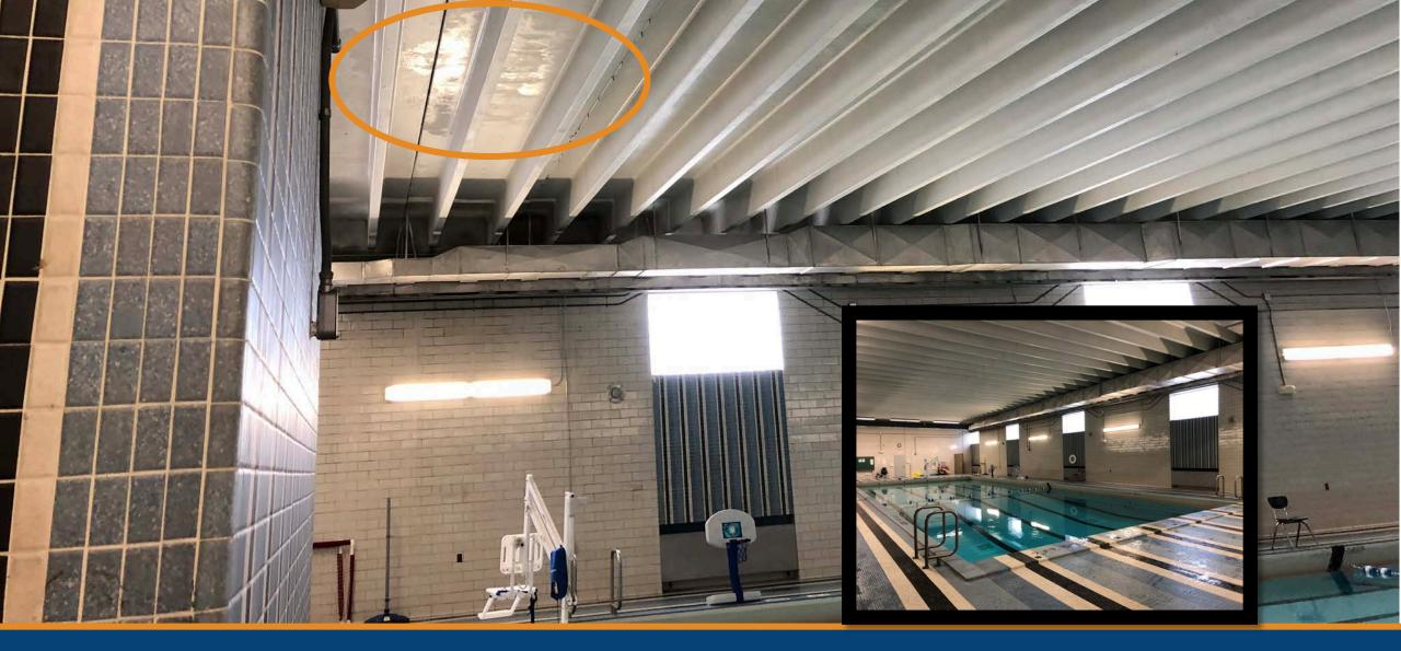
Condensation in pool due to faulty HVAC and saturated or insufficient roof insulation
