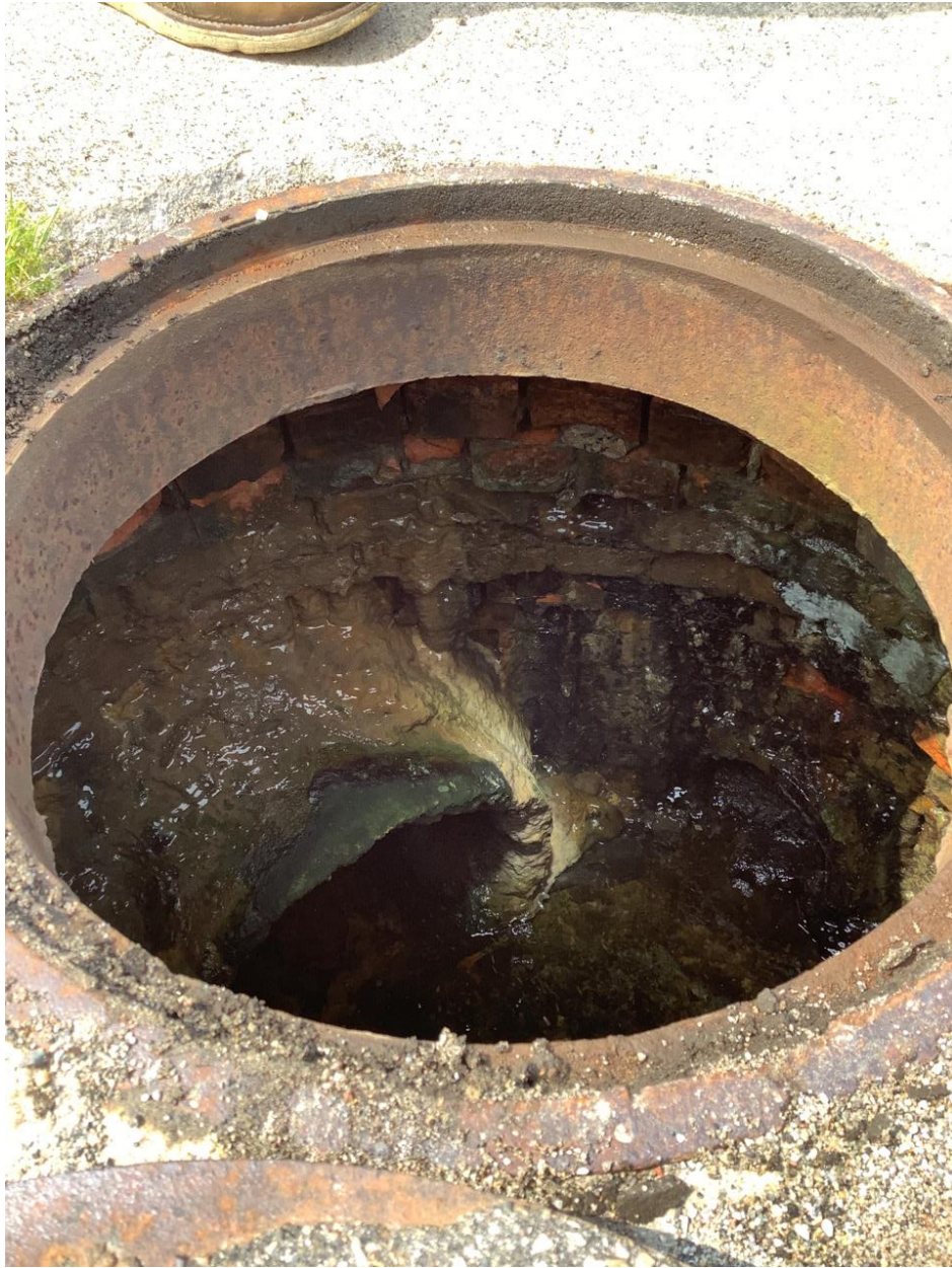
MHS26 – evidence of Infiltration into manhole – repairs needed
