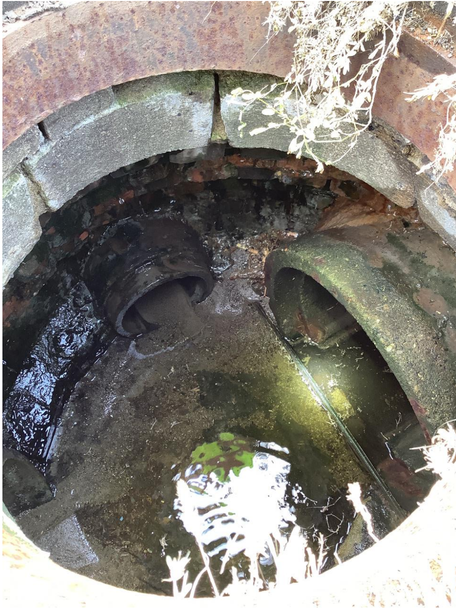
MHS22 – Evidence of Infiltration into manhole- repairs recommended
